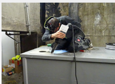
Building a tank in a small space
