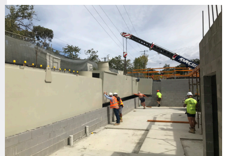
Welding modules together on site
