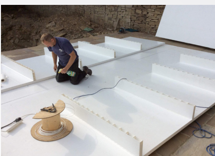
Pool welding on site
