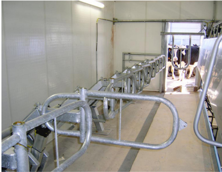
WALL CLADDING MILKING PARLOUR
