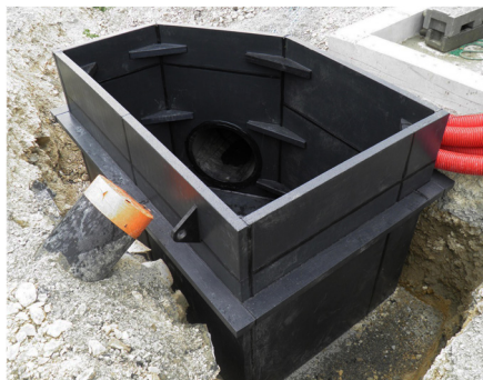
RAIN WATER TANK
