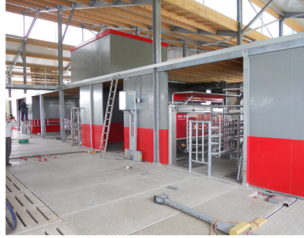
STATION DE TRAITE
