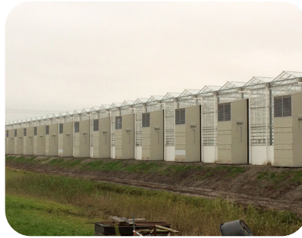
Heat recovery system
