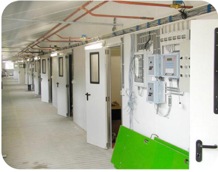
Corridor with interior doors and windows
